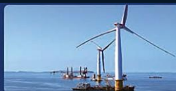
OFFSHORE WIND POWER Foundation Inspection
